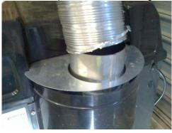
3/ Form extra bends where required. Care should be taken when forming bends to not create a low point where condensation may collect. Condensation should be able to drain to the heater or out the flue outlet. The flue should be bracketed at intervals of 1 M using standard 125 mm standoff brackets available at most plumbing suppliers.
